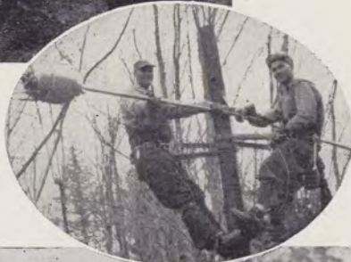
Controlling the cable guide and spinner at Livermore, Me., are Thomas McNeil and George A. Staples.
