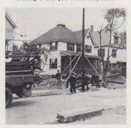
Falling trees and broken poles drop this cable onto the street at Melrose, Mass.
