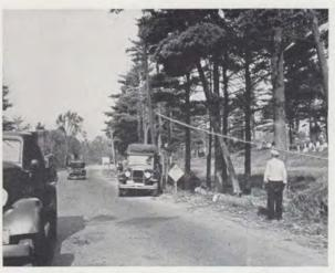
Truck pulls cable to position on a new pole at Spencer, Mass.
