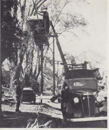
This cable crew from the Bell Telephone Company of Pennsylvania are at work near Wakefield, R. I. Notice the aerial ladder for cable work, one of the many kinds of Bell System equipment which were rushed into New England.
