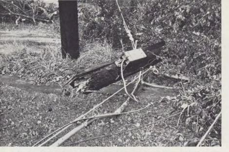
This pole could not stand the strain, so terminal box, cable junction, guy wire and pole tip crashed among broken branches on Main Street,
