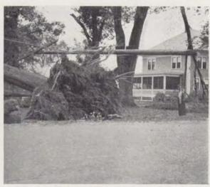
This cable on Main Street, Northfield, Mass., is suspending a telephone pole in mid-air, leaving only the stump in the ground.
