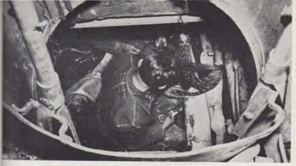
Splicer at Providence, R. I., who went down into flooded manboles to dry out our cables before the water had been completely pumped out.
