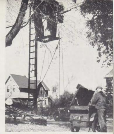
Cable splicers from the Bell Telephone Company of Pennsylvania working on a 720-pair toll cable in Wakefield, R. I.
