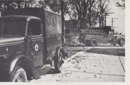
New England Telephone and New Jersey Bell Telephone Company trucks working together to repair burricane damage to cable line in Seekonk, Mass.
