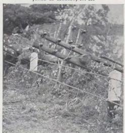
White plugs in Jacks at Keene, N. H., indicate the lines which were out of service. After the burricane only 50 of 1853 lines were working. This picture taken three days after the storm, shows bundreds of lines still out of order.
