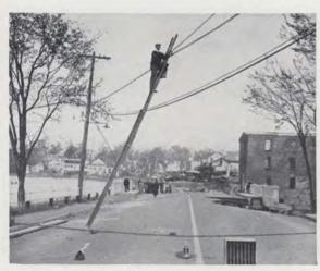
The Brookfields are again connected with the world as the first pair in a new cable is spliced in at East Brookfield, Mass.
