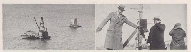
Left: The lighter out in the bay engaged in the work of laying the cable. Right: The field telephone connection on shore from which orders from the lighter were received. Supervising Foremen H. L. Buteau and W. J. Ryan (at the telephone) are keeping in touch
