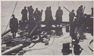
View on the deck of the lighter which was used in the laying of the cable in Mount Hope Bay. At the right may be seen the cable brakes which regulate the paying out of the cable.
