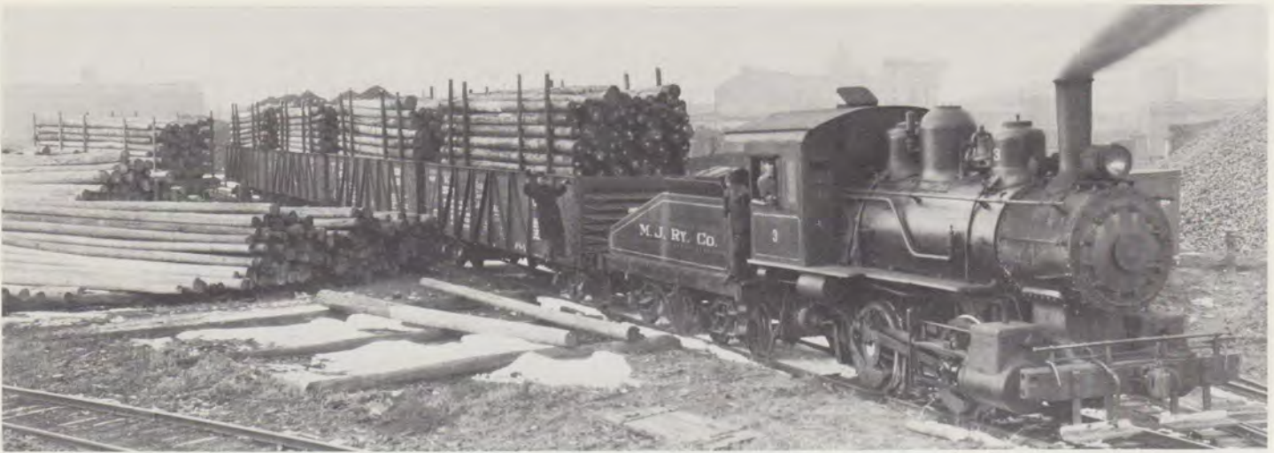
Telephone poles, treated at Hawthorne with a wood preservative, are hauled by the MJ on the first lap of their journey to Bell System telephone companies. Photo taken in 1925.
