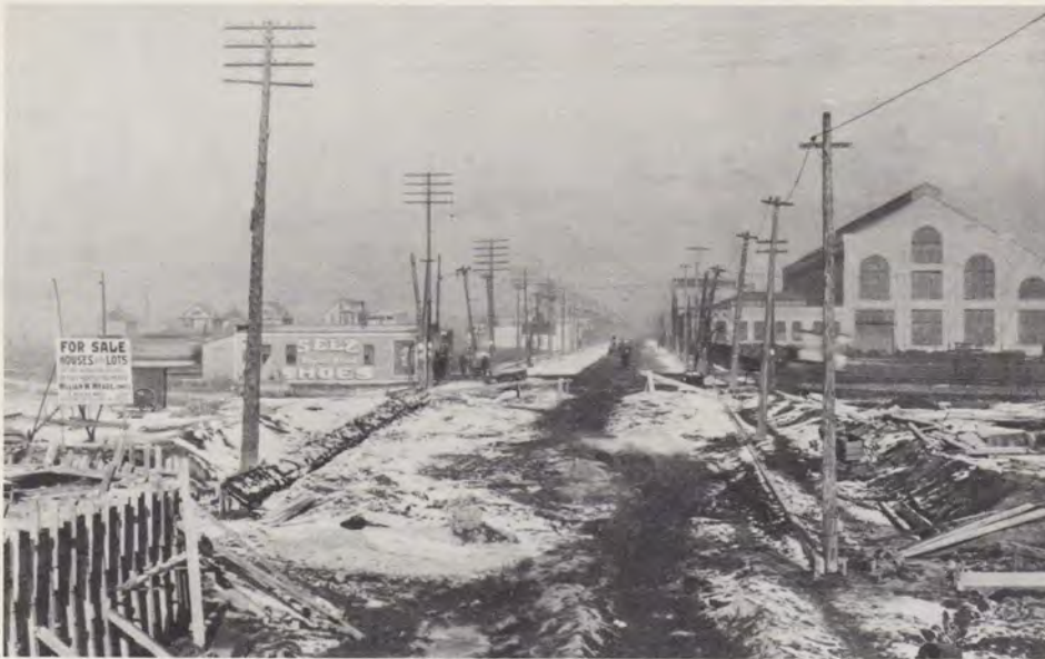
Cicero Avenue was a mess when this picture was taken in December, 1905, shortly after the Foundry building was completed.
