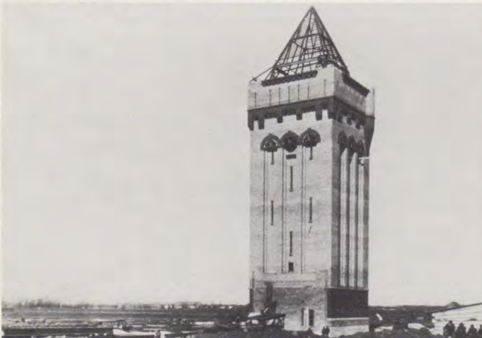
Hawthorne's water tower, completed in 1905, was the first structure built on the new property. It continues to stand, providing office space for fire control and security operations.
