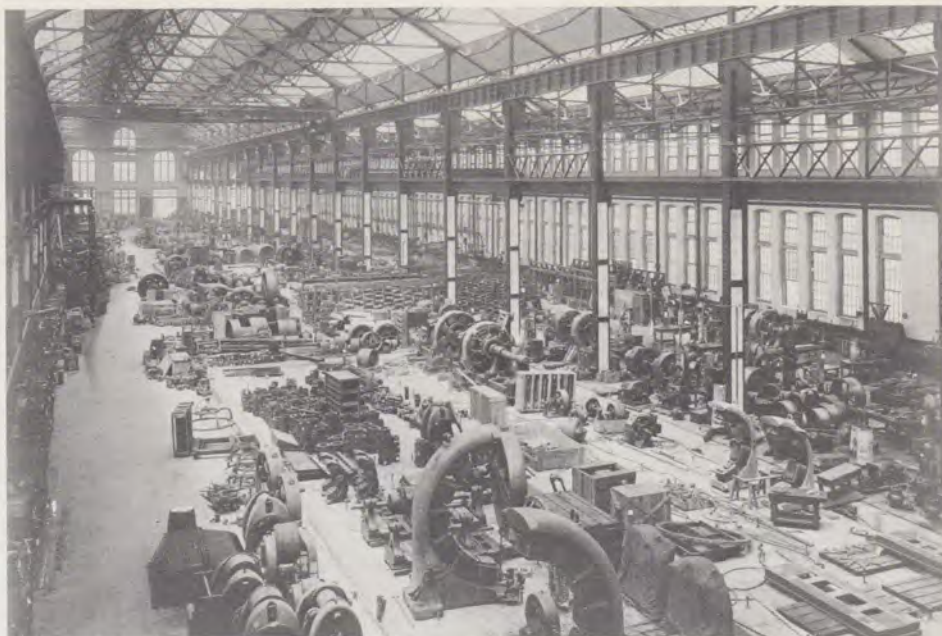
Hawthorne's Power Apparatus shop as it looked on July 8, 1905.
