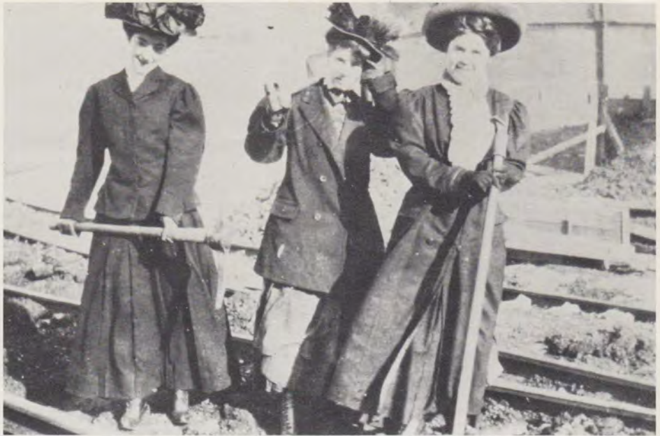
These Western Electric ladies were happy to give symbolic support to building tracks for the Manufacturers Junction Railway, the factory's main artery for moving raw materials in and completed cable out.
