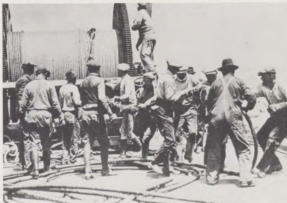
Pulling cable was literally a 'team' job when this photo was snapped about 1906. From the outset, telephone cable was a primary Hawthorne product.
