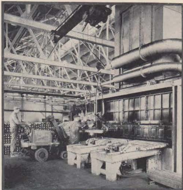
Left—Loading billets of copper in a modern heating furnace.
