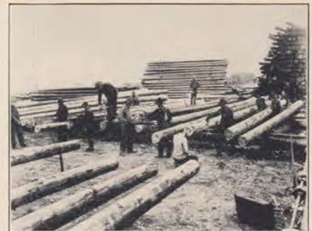
Prospective telephone poles are carefully inspected in a concentration yard for any possible flaws.
