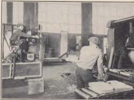
Taking the temperature of an ingot of aluminum alloy is very important if it is to be rolled still more to change its shape.
