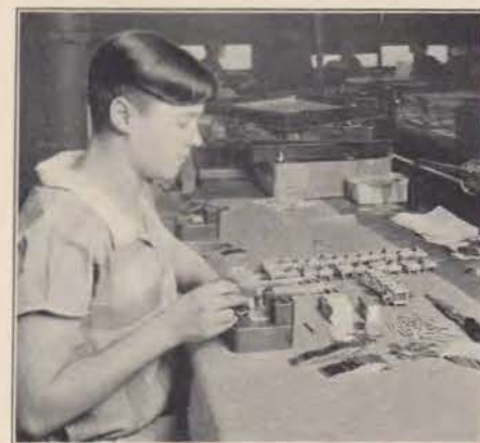
Thin sheets of mica are assembled for the condensers used in certain special telephone circuits which carry several messages at once over the same pair of wires.
