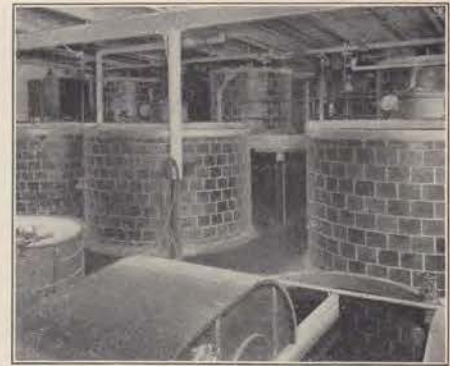
Storage tanks for pulp used in insulating cable wires.
