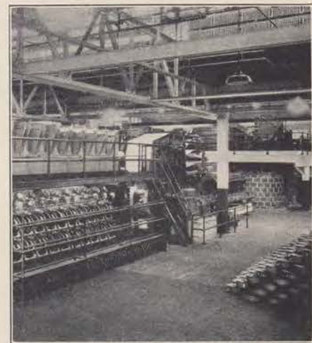
Equipment for applying paper pulp insulation to wire used in making certain types of telephone cable.
